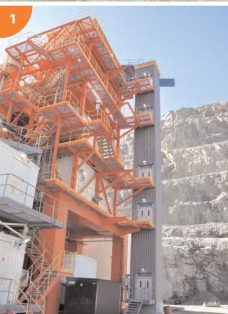
1 In-pit Crusher Elevator: ALIMAK SE 1000 Capacity: 1000 kg Lifting height: 24 m
