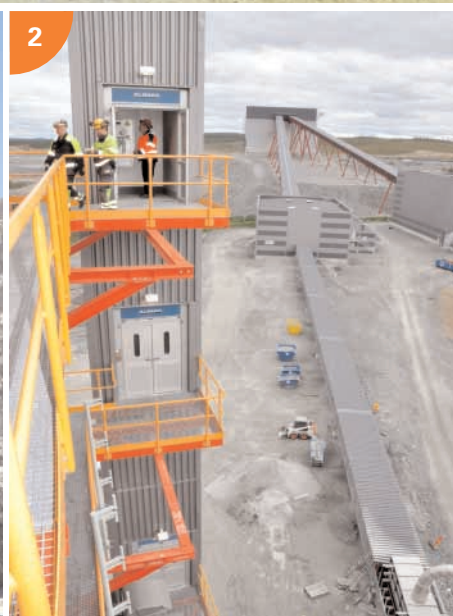
2 Surface Crusher Elevator: ALIMAK SE 1000 Capacity: 1000 kg Lifting height: 24 m
