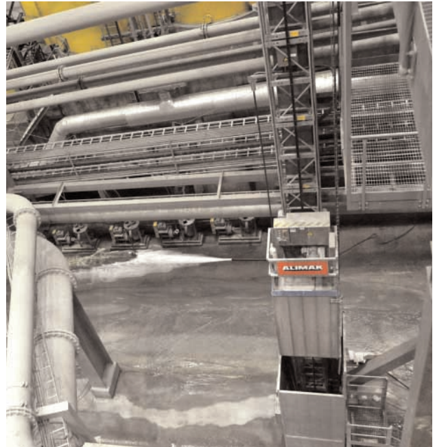
One out of the seven Alimak rack and pinion elevators working at the Aitik copper mine.
