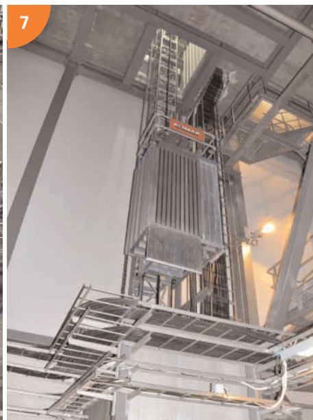
De-watering Elevator: ALIMAK SE 1000 FC Capacity: 1000 kg Lifting height: 18 m
