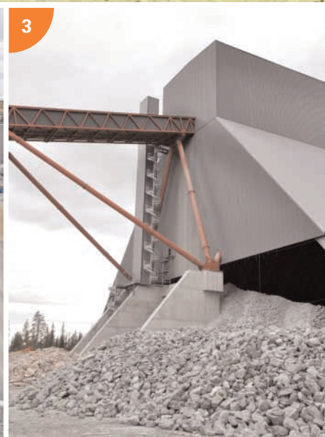
3 Ore stockpile Elevator: ALIMAK SE 1000 Capacity: 1000 kg Lifting height: 48 m
