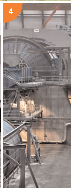
4 Grinding Elevator: ALIMAK SE 1000 Capacity: 1800 kg Lifting height: 18 m
