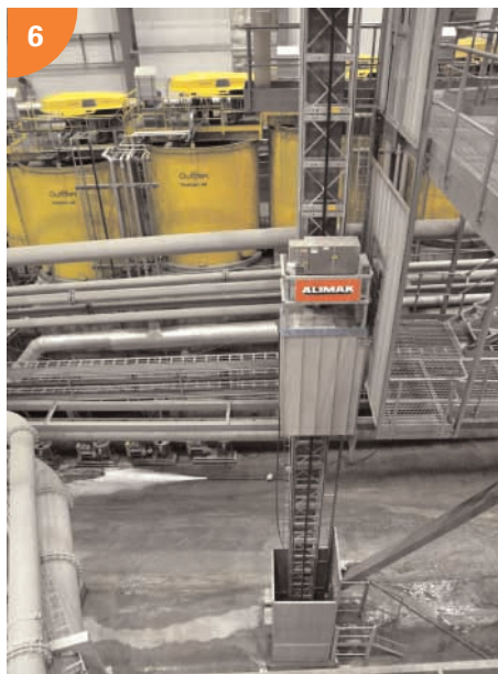
Flotation Elevator: ALIMAK SE 400 FC Capacity: 400 kg Lifting height: 14 m
