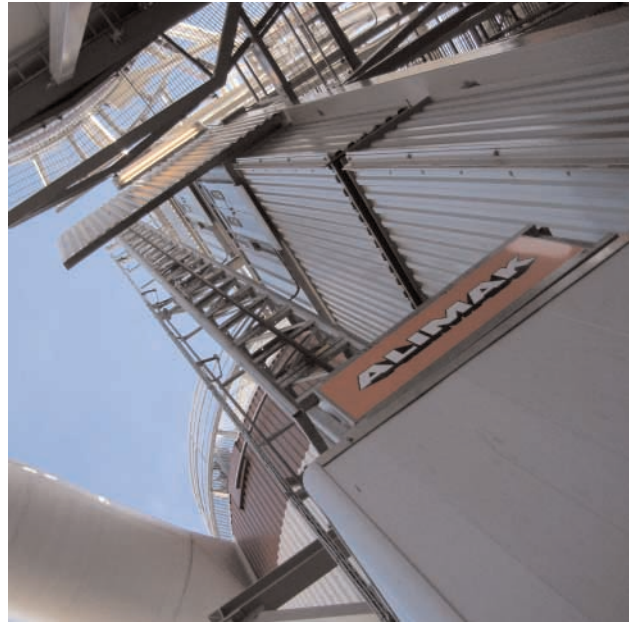
The Alimak elevator is being used frequently at Domsjö Fabriker.
